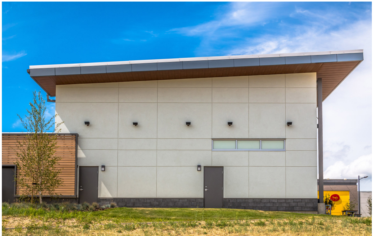
One of Several Feature Glass Gabion Walls
