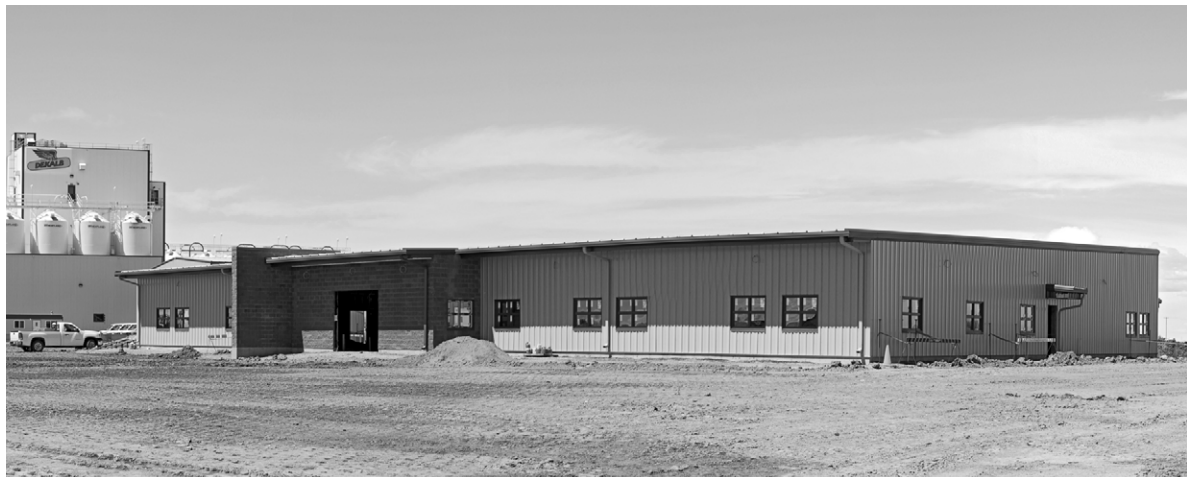
Completed Building Shell at Mid-Construction Term.
