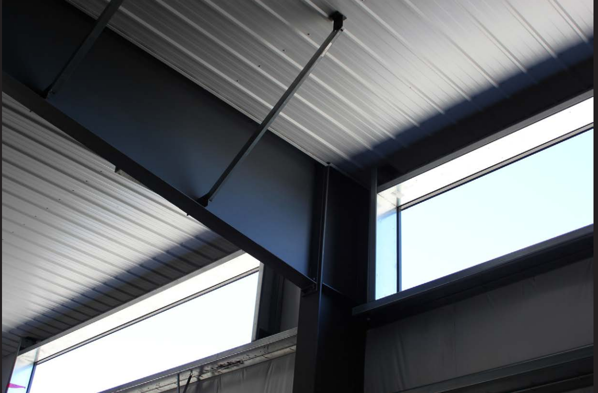
Exterior Building Views & Interior Building Structure
