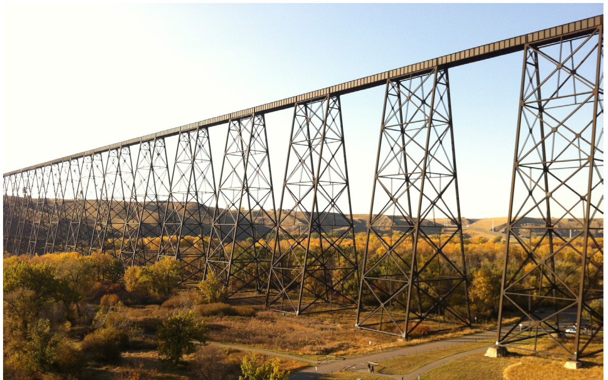
High Level Viaduct, Lethbridge, Alberta
