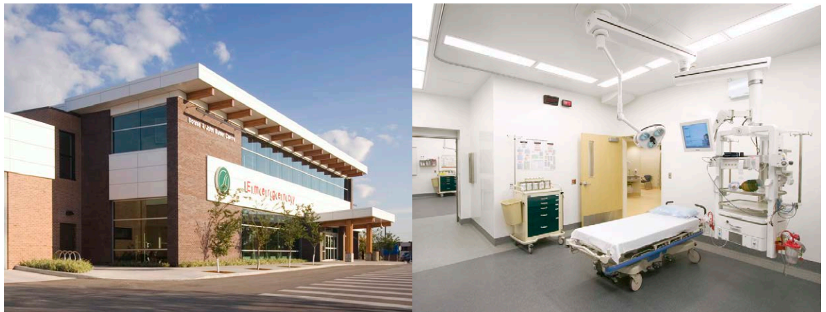
New Addition & Entrance, Trauma Room Facilities
